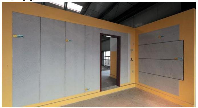
Compared with traditional internal wall partition materials, AAC internal panels have obvious advantages in various technical performances: lightweight, high strength, thermal insulation, fire resistance, sound insulation, seepage prevention, frost resistance, durability, anti-seismic, high softening coefficient, no radiation, good creativity, scientific installing method, convenient and quick construction.
