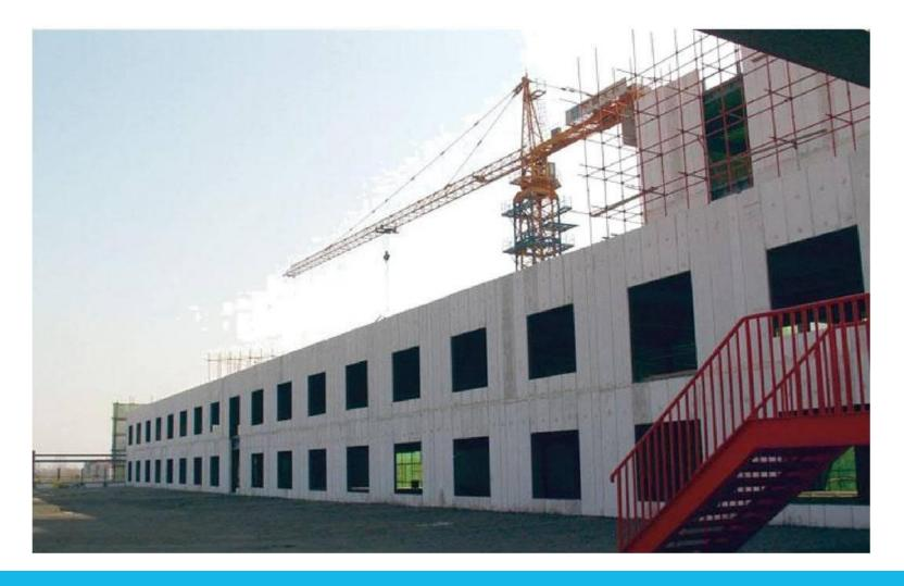
AAC panels improve the reliability and security of node strength in external walls. During the rotation and extension in plane of the connecting nodes of wall panels, AAC panels ensure that the walls can be adapted to the interlayer displacement in different directions of the main structure, and satisfies the need for the interlayer deformation of the main structure conforming to the seismic design intensity.
