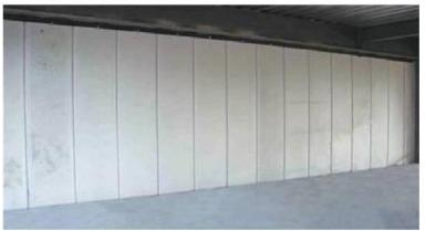
AAC internal panels are reinforced by antirust double-layer and two-way steel mesh. They have good load-bearing capacity, the static hanging weight in a single point being 120kgs. They are produced in high temperature, high pressure and steam curing, with the minimum shrinkage ratio in the inorganic materials, caulked with special polymer binders, which can effectively prevent cracking.
